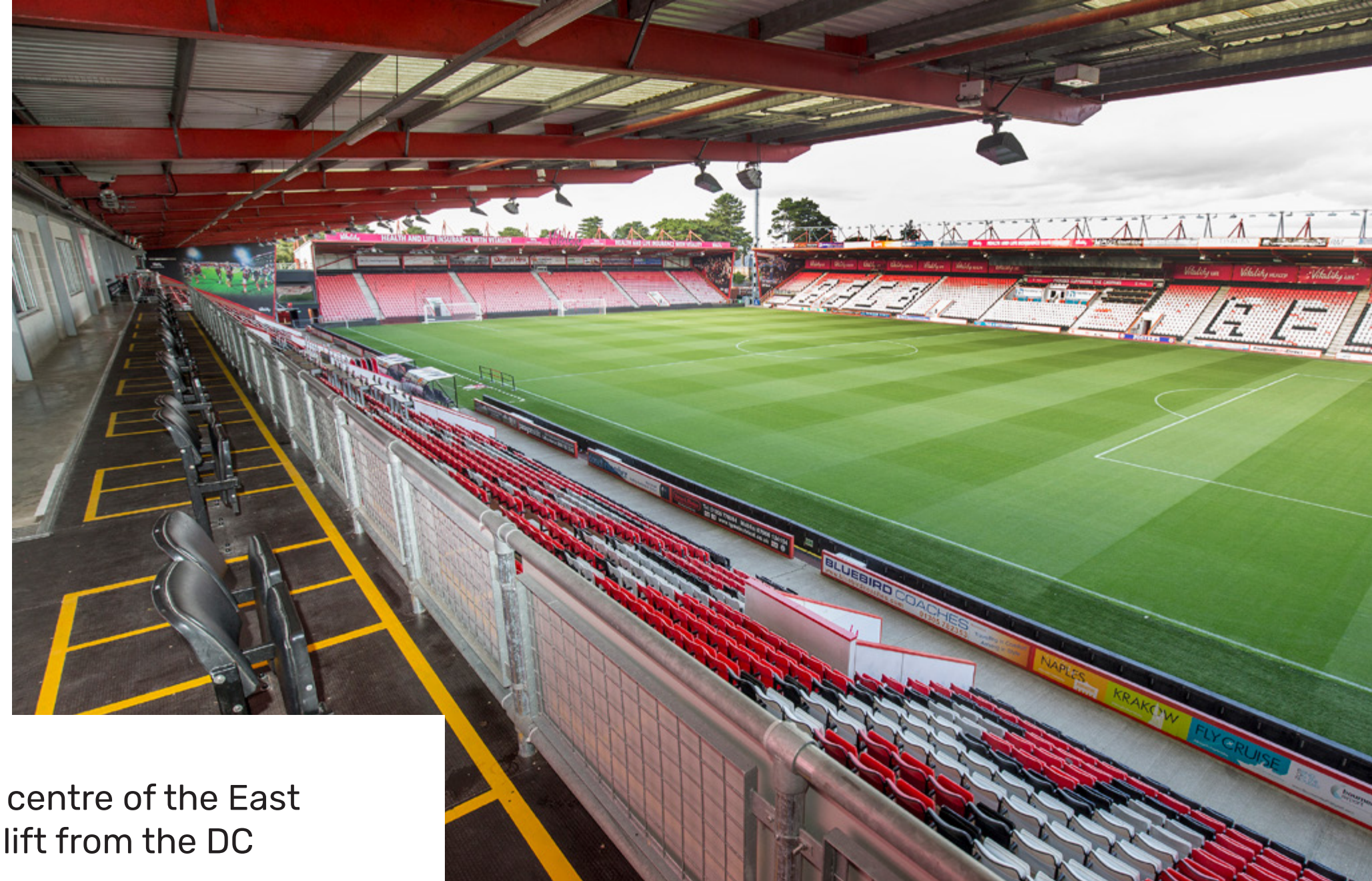
Photo: Main Stand Raised Viewing Platform
