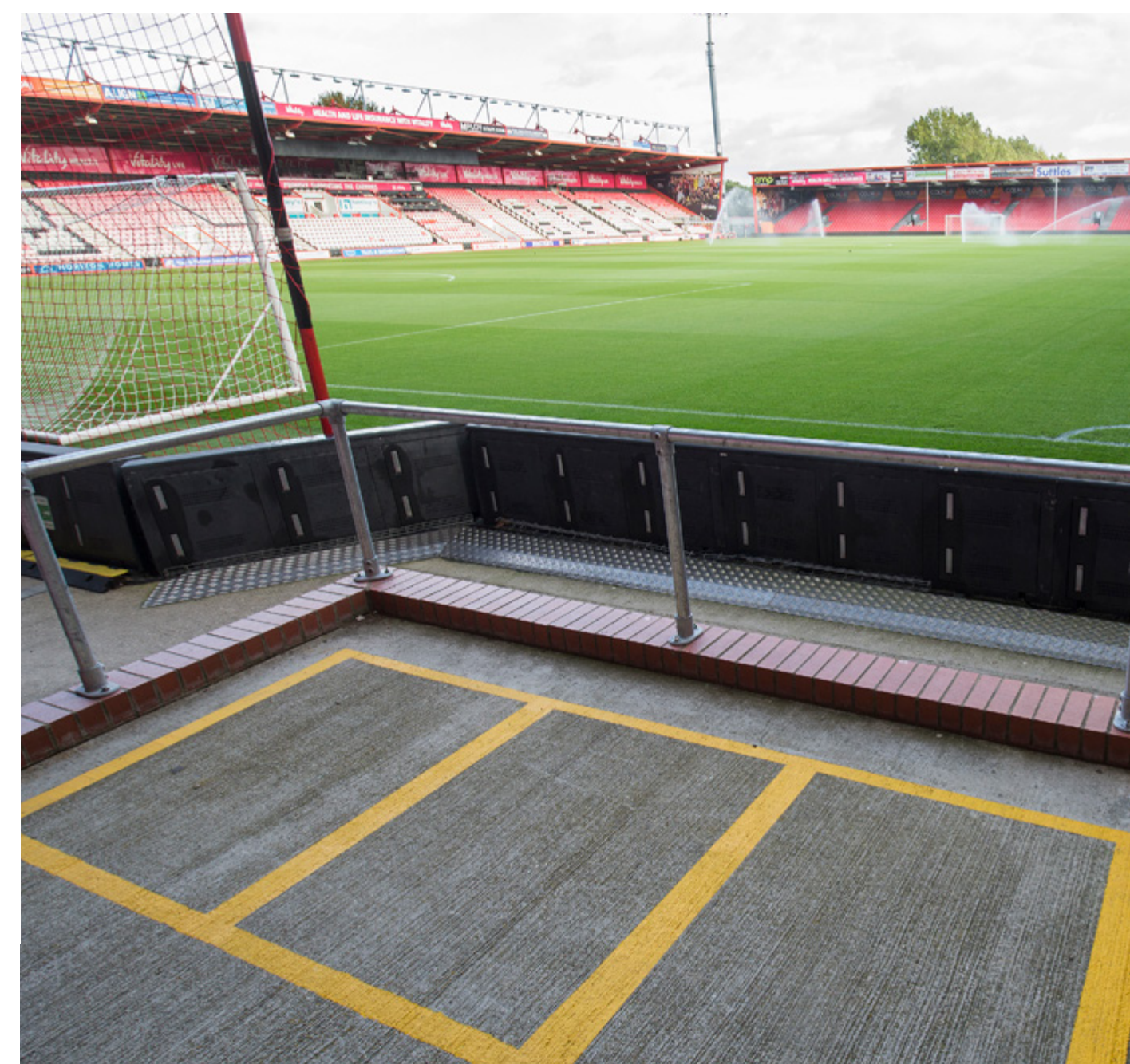
Photo: North Stand Viewing Platform
